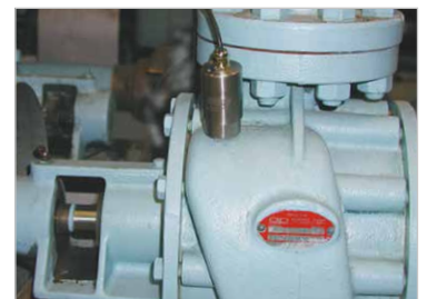
Monitor cavitation, bearings, and valves
